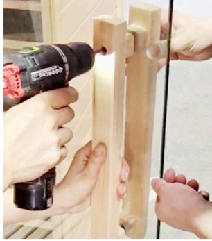
Door Handle Installation
