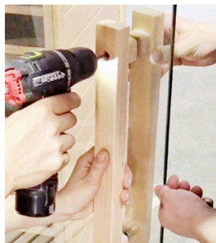
Door Handle Installation
